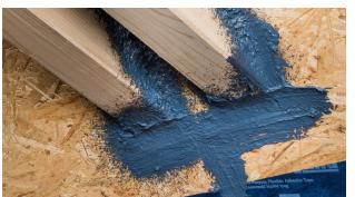
9. The finished joint at a double collar tie penetration
