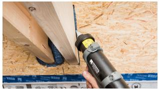
**5. Fill the joint** Fill the joint with a sufficient amount of AEROSANA VISCONN / FIBRE.
