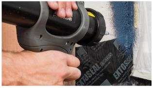
**8. Interior and exterior use** AEROSANA VISCONN / FIBRE can be used for interior and exterior window joints. The installation method is identical in both cases.
