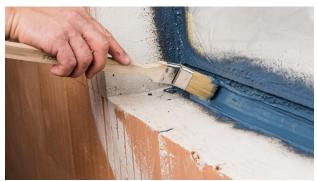
7. Check the joint If necessary, seal any gaps with a brush and AEROSANA VISCONN / FIBRE.
