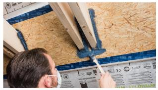
**8. Check the joint** If necessary, seal any gaps with a brush and AEROSANA VISCONN / FIBRE.
