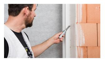
**3. Cut away any excess insulation material** If necessary, cut away any protruding insulation.
