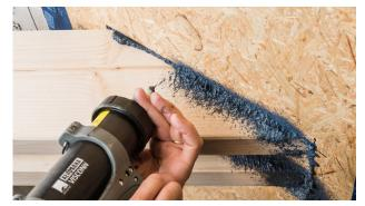
**6. Spray over the joint** Set the AEROFIXX to spray application and spray over the joint in a generous manner.
