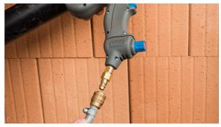
**6. Connect AEROFIXX** Connect the spray gun to the compressed air. Air requirement approx. 250 I/min. Set the pressure to 6 bar (87 psi) on the pressure reducer.
