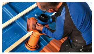
10a. On slightly slanted roofs: Joint at pipe feed-throughs
