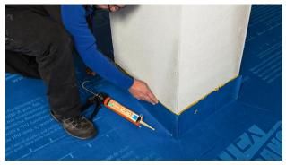
12b. On slightly slanted roofs: Joints with protruding building components (e.g. chimneys)
