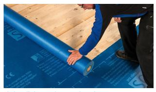
2b. Install the membrane and overlap
