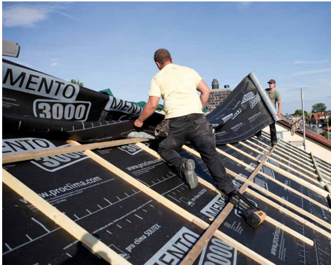
Fig. 1: A modern roofing underlay membrane as an external sealing layer underneath the subsequent roof covering.
