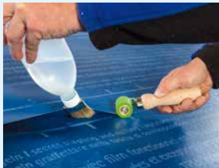
Fig. 20: Welding of underlay membranes: The functional layers of overlapping membranes are welded together homogeneously with a solvent welding agent or a hot air gun.
