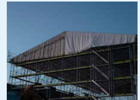
Fig. 3: A temporary shelter over a roof.
