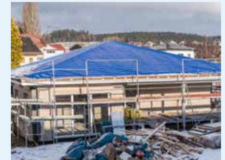
Fig. 2: Tarpaulins covering a roof.
