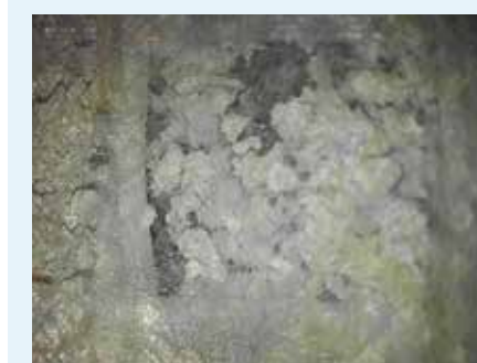
Fig. 35 a/b: Microscope images of underlay membranes showing crack formation and serious degradation after 13 weeks of outdoor exposure.
