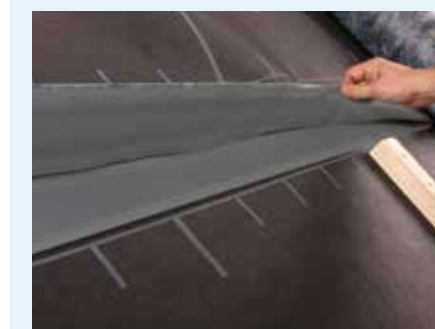
Fig. 41: Membrane overlaps with self-adhesive strips – in this case, the adhesive bond is located under the overlap and is protected against water run-off. The adhesive-to-adhesive bond is reliable even under unfavourable conditions.
