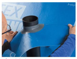
**2. Create the bond**Guide WELDANO ROFLEX PLUS over the pipe.
