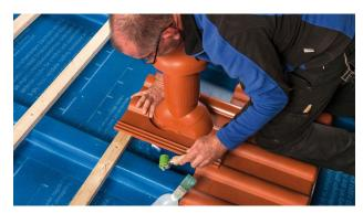
10b. On slightly slanted roofs: Joint at pipe feed-throughs
