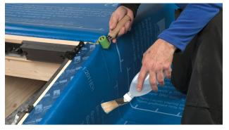
**25.** Weld the layers of SOLITEX WELDANO 3000 to one another on the sides.
