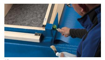
Fold the excess pieces and weld them to the lower membrane. Pay particular attention to ensuring the corners are sealed tight.
