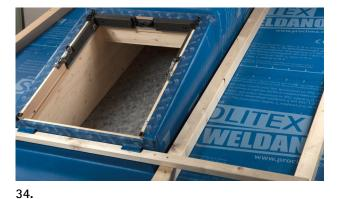
Install the counter battens and horizontal roof battens, and screw the mounting brackets into place. You're finished!
