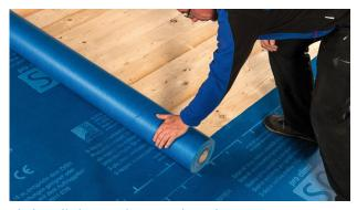
2b. Install the membrane and overlap
