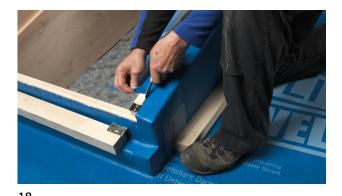
Cut to size parallel with the window frame. An auxiliary batten can be used to help affix the lower edge without folds or creases.
