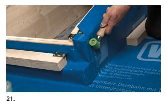
Press down on the welded bond (e.g. using a pro clima ROLLFIX silicone roller).
