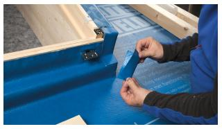
**31.** Remove the auxiliary roof batten and cut out fitting pieces for sticking over the mounting brackets.
