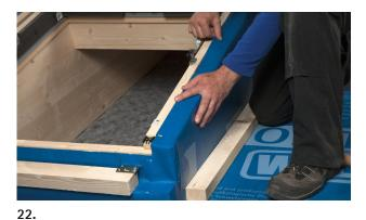
Stick SOLITEX WELDANO 3000 onto the edge of the frame. Put the membrane in place on the adhesive bed, leaving slack to allow for expansion. Do not press the adhesive completely flat so as to allow for relative motion between components.
