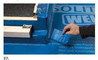
To cover the cut edges in the corner area, cut out a small strip of SOLITEX WELDANO 3000 and put it in place.
