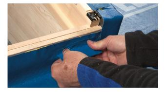
**32.** Enclose the mounting brackets by means of welded bonds.
