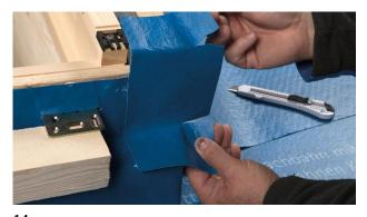
**14.**Cut into the fitting piece horizontally at the two edges. Do not cut right up to the frame, but instead leave a few millimetres of material in place to seal the corner.
