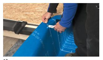
Guide the membrane from the main surface onto the side of the wedge-shaped frame. Alternatively, cut a new strip of SOLITEX WELDANO 3000, guide it up along the wedge-shaped frame and weld it at the bottom to the flat membrane.
