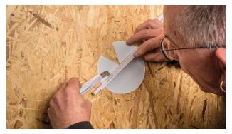
2. Cut to size Place the measuring rule on the installation edge and cut TESCON TANGO to size.
