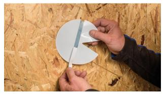
**1. Prepare the corner patch** Pre-fold TESCON TANGO and partially remove the release film of the attachment surface.
