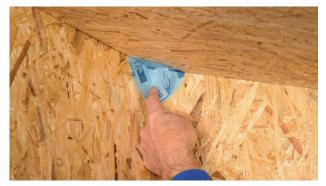
**4. Rub the patch firmly into place** This step can be carried out in a manner that is kinder to your hands by using the pro clima PRESSFIX application tool.
