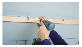
9a. Detail solution for blown-in insulation material
