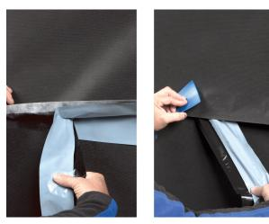
**3. Stick overlaps using 'connect' adhesion technology** Stick membrane overlaps in the case of 'connect' membranes with two integrated self-adhesive strips. Rub the resultant adhesive joint firmly using the pro clima PRESSFIX. Ensure that there is sufficient resistance pressure.
