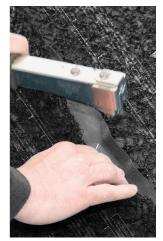
9. End joint: Align the membrane and fasten it in place
