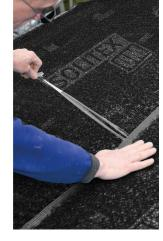
Clean the subsurface (dry and free of dust, silicone and grease) and carry out an adhesion test, if necessary. Lift up the second membrane, remove the release film and gradually stick the membranes in place using the integrated self-adhesive strips, ensuring that there are no folds or tension. Rub the adhesive joint firmly.
