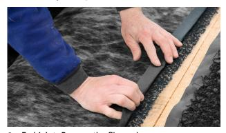
8a. End joint: Remove the fibrous layer
