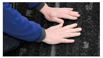
**7.** Rub firmly to secure the adhesive bond Rub the adhesive joint firmly.
