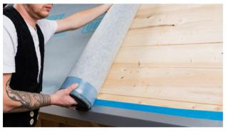
12. Installation of the membranes onto wood sheathing
