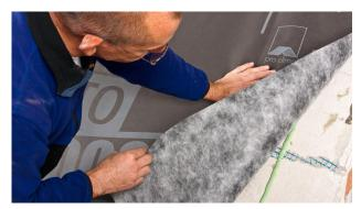
7b. Sealing to rough or mineral subsurfaces
