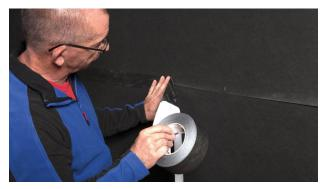
5a. Alternatively: Taping over the overlaps with TESCON INVIS
