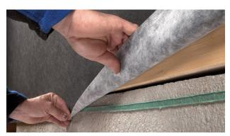
7. Alternatively: Sticking to rough or mineral surfaces (e.g. floorboard) with CONTEGA MULTIBOND
