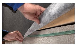
7. Alternatively: Sticking to rough or mineral surfaces (e.g. floorboard)
