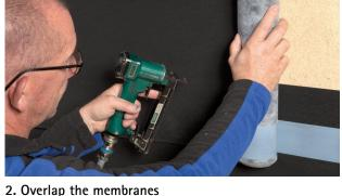
Clean the subsurface (dry and free of dust, silicone and grease). Overlap the membranes by approx. 10 cm (4") so that they are watertight. The printed markings on the membrane serve as a guide here.
