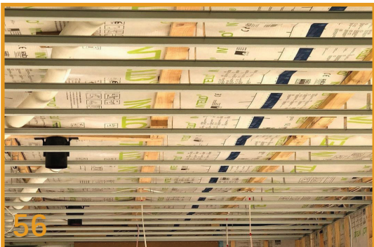
Fix INTELLO® PLUS with Service Cavity Ensure all laps, connections and penetrations are taped and sealed.
