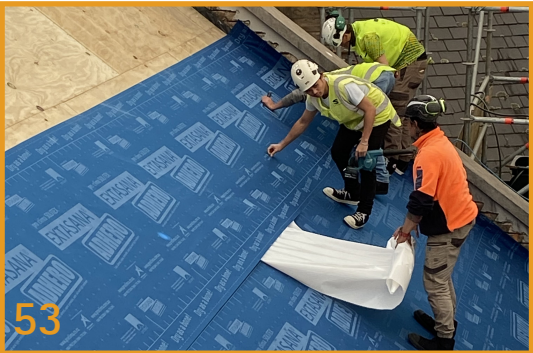
Place and Adhere Course by Course The membrane may be rolled out course by course on roofs above 5° pitch.
