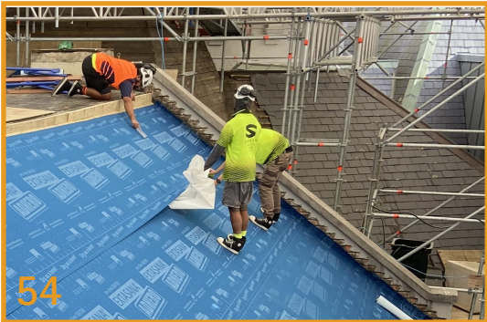
Overlap, Remove Backing and Adhere Overlapping joints by 150 mm, remove backing and adhering in same method as for low pitch roofs.
