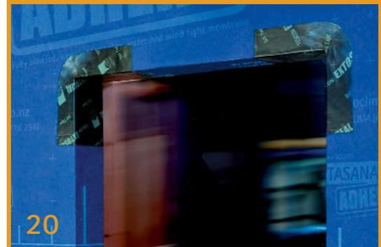
**Seal Exposed Framing at Top Corners**
