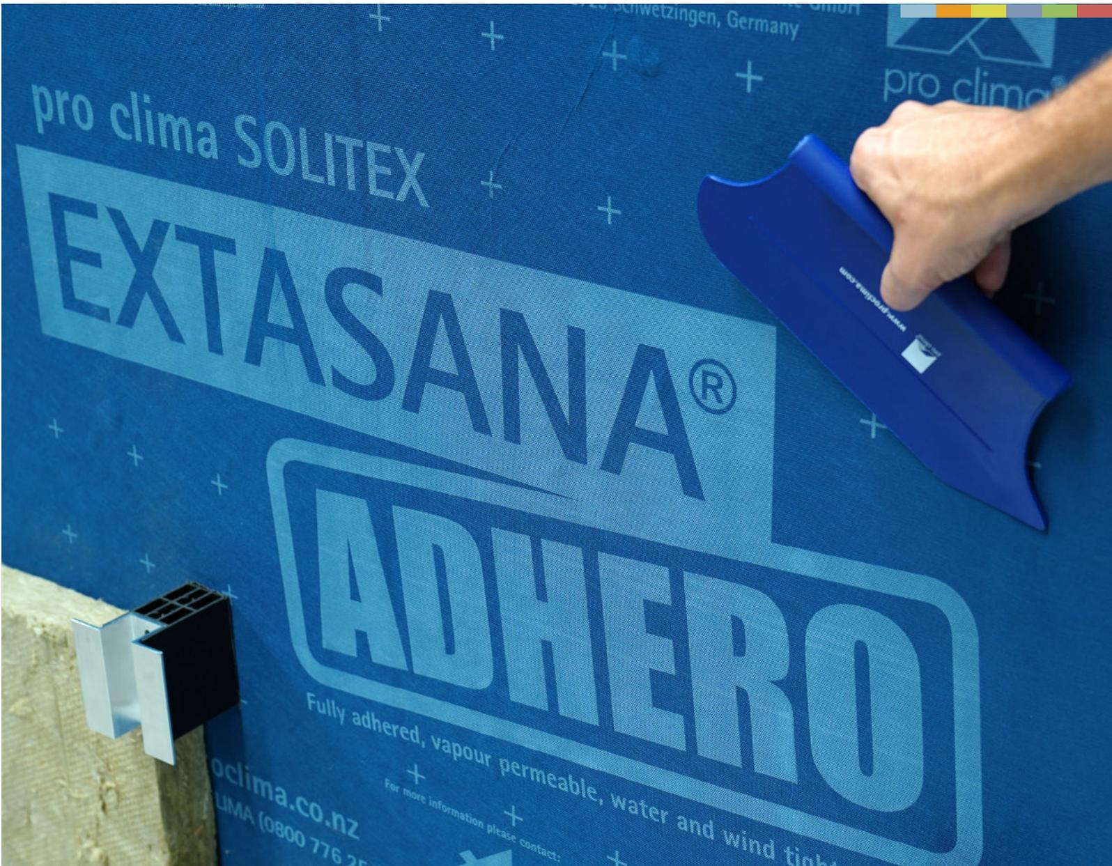
Self-Adhesive Weather Resistive Barrier for Walls and Roofs
