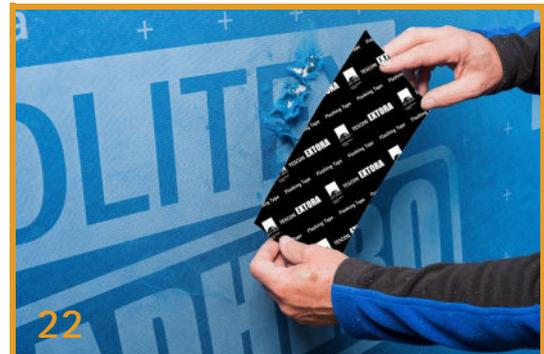
**Repair Abrasions Using TESCON EXTORA®**
