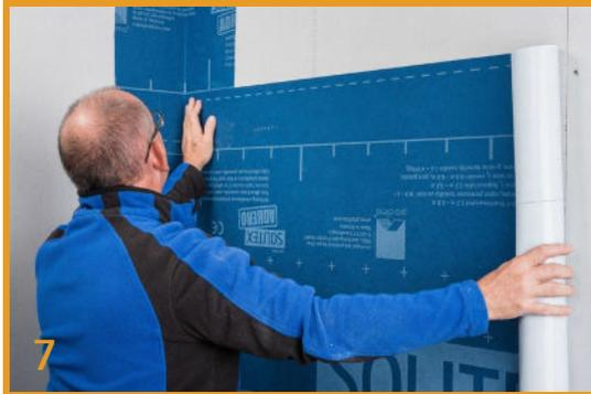
**7 Apply Membrane to Align with Internal Corner**
