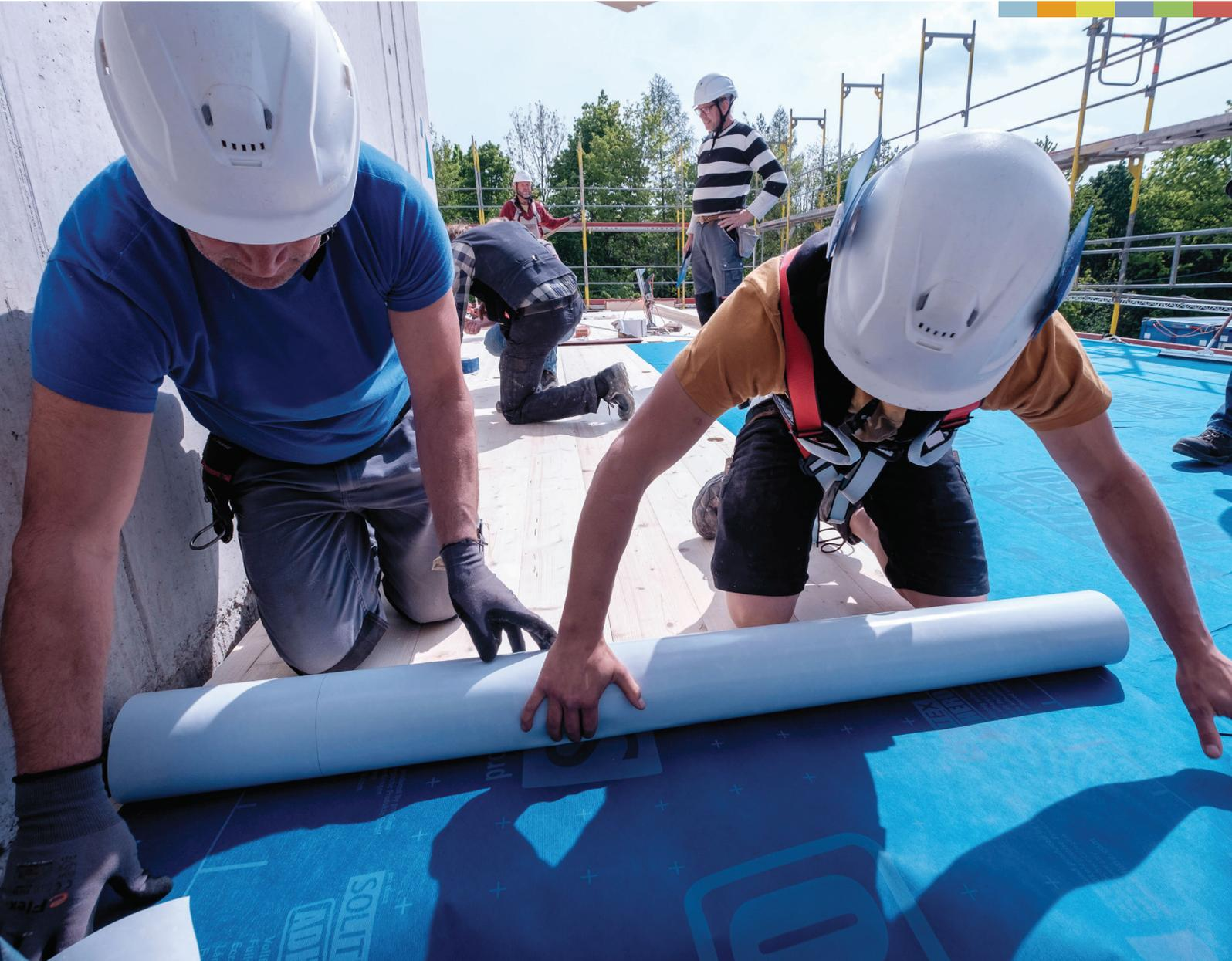
Self-Adhesive Weather Protection for Walls and Roofs
