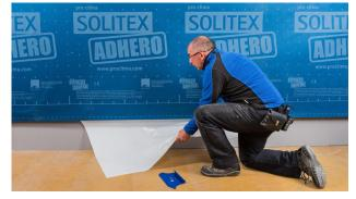
**10. Remove the remainder of the release film** Grip the wide release film by the previously folded corner and pull it off.
