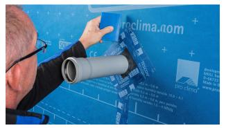
**22. Pipe feed-throughs with ROFLEX** Seal pipe feed-throughs with a suitable ROFLEX grommet. Stick the grommet to the subsurface using TESCON VANA. Rub over the taped surface using PRESSFIX XL.
