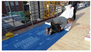
**5. Stick the surface** Roll out the membrane along the marking and gradually stick it to the subsurface.
