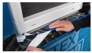
18. Seal window joints on the inside and outside
