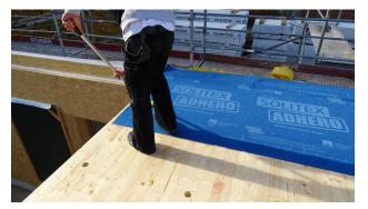
**6.** Rub the membrane firmly to secure the adhesive bond Rub the membranes firmly into place – e.g. using a brush or PRESSFIX XL.
