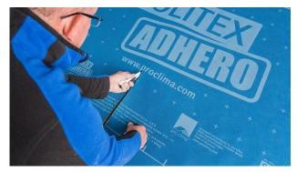
**4. Cut the membranes** Cut the membranes down to the required length. There are markings to make your work easier.
