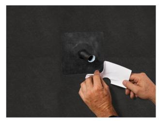
2. Remove the release paper Remove the release paper around the pipe/cable feed-through.
