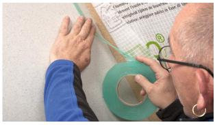
2. Apply a line of adhesive Position ORCON MULTIBOND on the subsurface to be bonded, roll it out and gradually stick it to the subsurface.
