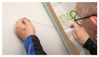
**3. Remove the release film** Gradually remove the release film.
