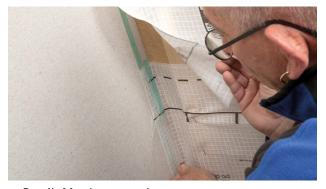
**5. Detail: Membrane overlap** Stick membrane overlaps together using ORCON MULTIBOND; press the membranes firmly together using PRESSFIX.
