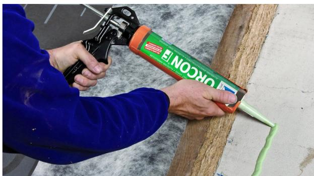
**7a. Sealing to rough or mineral substraces**
