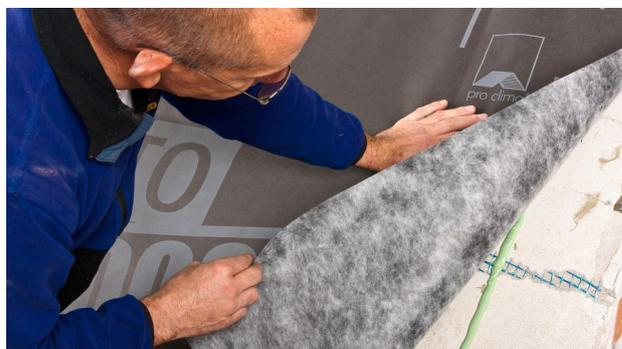
**7b. Sealing to rough or mineral substraces**
