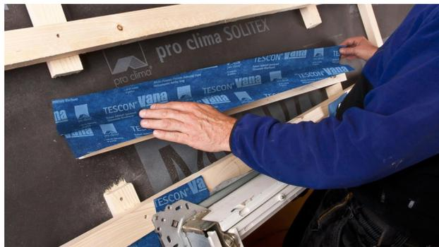
**9. Installation of a water deflector**
