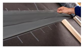
**4a. 'connect' adhesion** Sticking of membrane overlaps using 'connect' membranes with two integrated self-adhesive strips.
