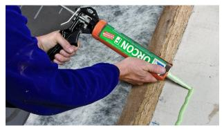
**7a. Sealing to rough or mineral subsurfaces** First create a smooth finish on rough wall caps. Clean the subsurface. Apply a line of ORCON F adhesive sealant with a thickness of at least 5 mm (3/16") (more in the case of rough subsurfaces, if necessary).
