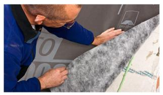
**7b. Sealing to rough or mineral subsurfaces** Apply the membrane, leaving slack to allow for expansion, and do not press the adhesive completely flat.
