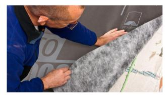
7b. Sealing to rough or mineral subsurfaces
