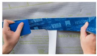
**5b. Rub the taped joint firmly** Rub the tape firmly using the pro clima PRESSFIX to secure the adhesive bond. Ensure that there is sufficient resistance pressure.
