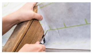
**5a. Joints at rafters** Cut the membrane as necessary and guide it around the rafters.
