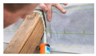
**5b. Joints at rafters** Bond the membrane to the top and sides of the rafters and to the ring beam using ORCON F.
