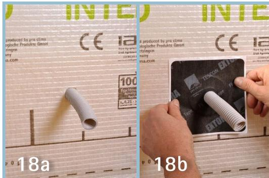
**For small pipes use ROFLEX 20 grommet**
