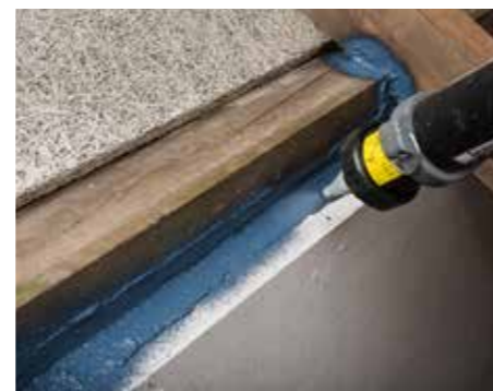
... for challenging refurbishment situations.
