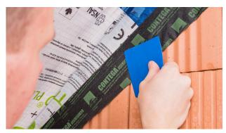
10. Masonry gable end wall, creating an airtight joint
