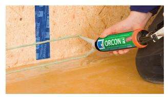
1. Joint between OSB wall and ground slab with INTELLO conneX
