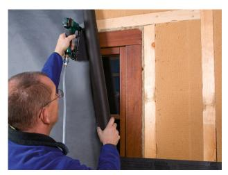
**8a. Sticking to windows** Install membranes continuously over window openings and attach them all around the window using a stapler. Then cut open the opening using a utility knife.
