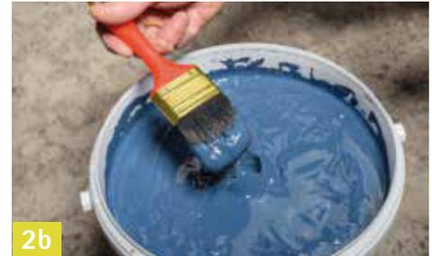
detected during spraying, these can be covered over with pro clima WYFLEXA fleece. To do this, paint AEROSANA VISCONN onto a piece of fleece, apply the fleece to the defect and spray over it.
