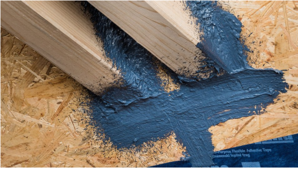
9. The finished joint at a double collar tie penetration Window joint with AEROFIXX
