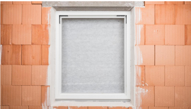
1. Initial situation Window is installed, window joint has been filled with insulation material.
