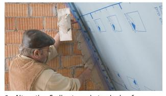
**8c. Alternative: Sealing to unplastered subsurfaces** First plaster behind the tape, then apply the tape to the wet plasterwork and plaster over it fully.
