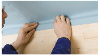
8b. Sealing to roughly sawn timber
