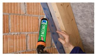
**8a. Alternative: Sealing to unplastered subsurfaces** Attach the CONTEGA PV plaster-sealing tape to the wall initially at discrete points using ORCON F. The adhesive strip should be facing inwards.
