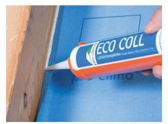
**6b. Seal at the rafters in an airtight manner** Apply a line of ORCON F adhesive sealant of at least d = 5 mm (3/16") to roughly sawn rafters, or more in the case of very rough subsurfaces if necessary, and stick the membrane to this.
