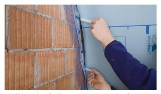
**8b. Alternative: Sealing to unplastered subsurfaces** Guide the vapour control membrane into position, remove the release film from CONTEGA PV and stick the vapour control membrane to the tape.
