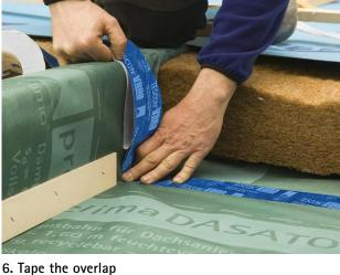
Clean the subsurface (dry and free of dust, silicone and grease) and carry out an adhesion test, if necessary. Centre the TESCON VANA system adhesive tape on the overlap and gradually stick it in place, ensuring that there are no folds or tension. Rub firmly using the pro clima PRESSFIX application tool to secure the adhesive bond. Ensure that there is sufficient resistance pressure.
