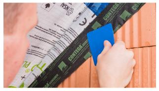
A - Transition between membranes and masonry wall
