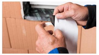
**3. Remove the first release film strip** Remove approx. 5-10 cm (2" - 4") of the narrow release film strip.
