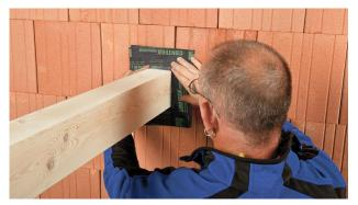
Cut the PRESSFIX tool as required to facilitate even pressing, and then rub
