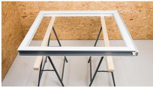
1. CONTEGA SOLIDO IQ is to be applied before the window is installed The frame is laid out flat.
