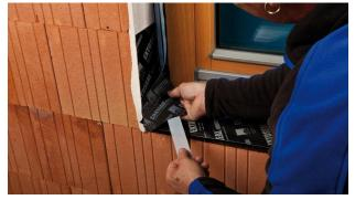
**5. Stick to the sub-sill flashing** Put the tape in position on the sub-sill flashing and stick it in place.
