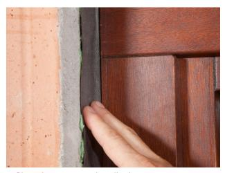
4. Place the tape onto the adhesive
