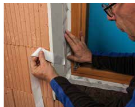
Stick onto the reveal and rub into place
