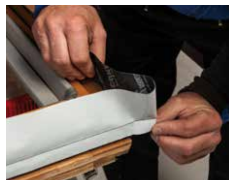
Preparation of corners
