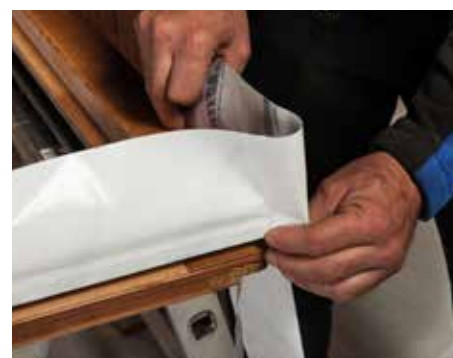
Preparation of corners
