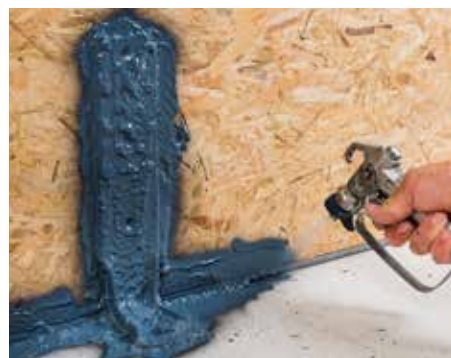
Airtight spraying over angle brackets,
