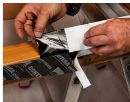
Stick the tape all around the window frame
