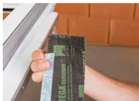
Remove the release film strip.
