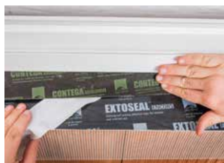
Install the window, remove the release film strip and stick the tape all around the window.
