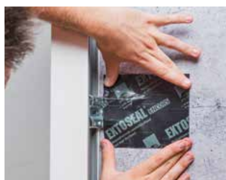
Waterproof taping of angle brackets.
