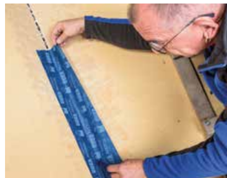
Tapes can be stuck directly onto recently applied primer.
