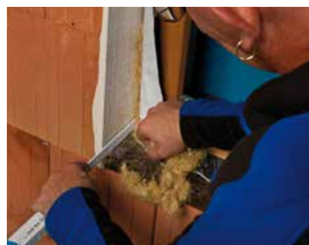
Install the window and insulate the joint
