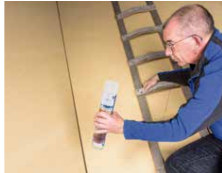
Use on wood-fibre underlay panels
