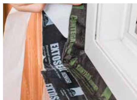
Stick to be airtight or resistant to driving rain in the corners.
