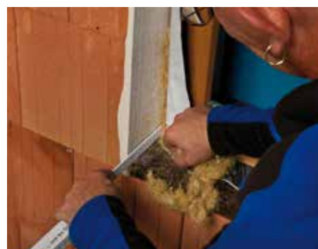
Install the window and insulate the joint
