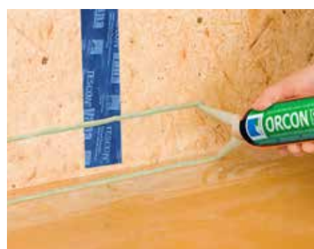
... and floor joints with wood-based panels,
