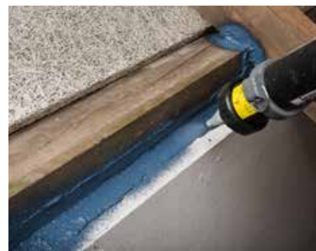
... for challenging refurbishment situations.
