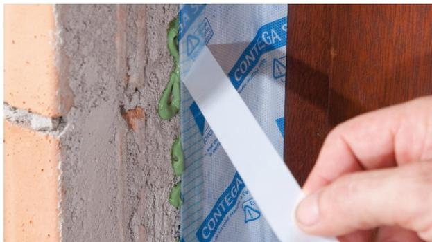
**3g. Remove the outer release film**
