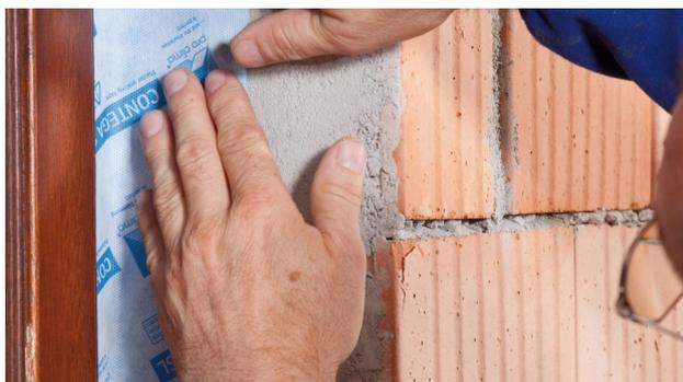
**4d. Place the tape onto the adhesive**
