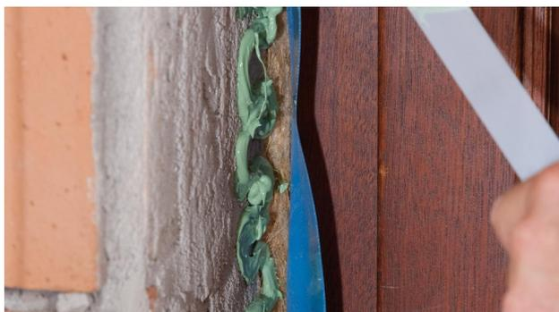
**4b. Remove the inner release film**
