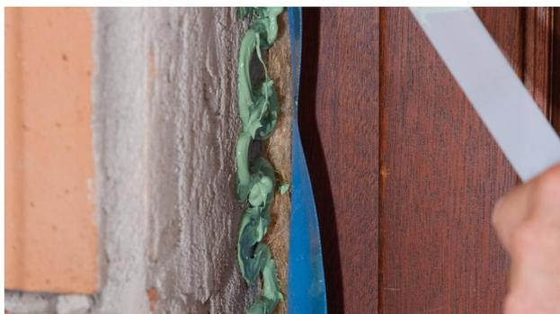
**4b. Remove the inner release film**
