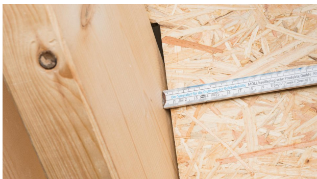
3. Check the joint width
