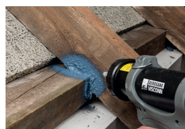
Sealing of penetrations on the interior or exterior
