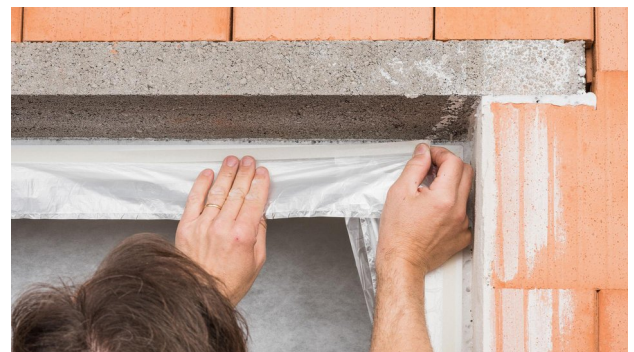
4. Apply masking tape to the window frame When doing this, leave a strip with a width of at least 6 mm free on the frame for subsequent sealing using AEROSANA VISCONN / FIBRE. Alternatively, remove the joint insulation to a sufficient extent to create a clean surface for a lateral bond to the side of the window frame.
