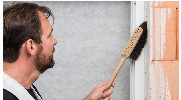
2. Preparation Brush off subsurfaces; if necessary, clean with a vacuum cleaner and wipe down.
