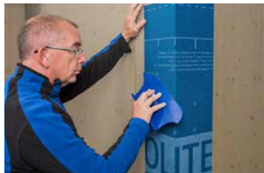
PRESSFIX XL Can be used to press SOLITEX ADHERO 1000/3000 into place easily and quickly
